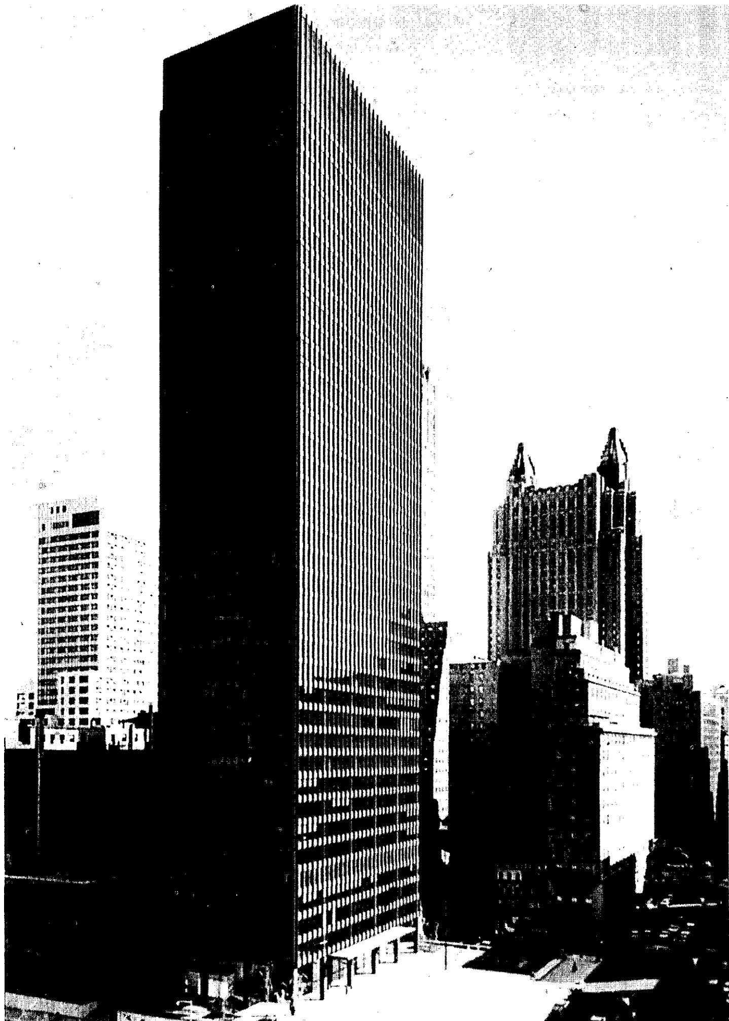
The Seagram building in New York, designed by Mies van der Rohe. Since the 1950s city centres all over the world have been filled with replicas of this 'International Style'
